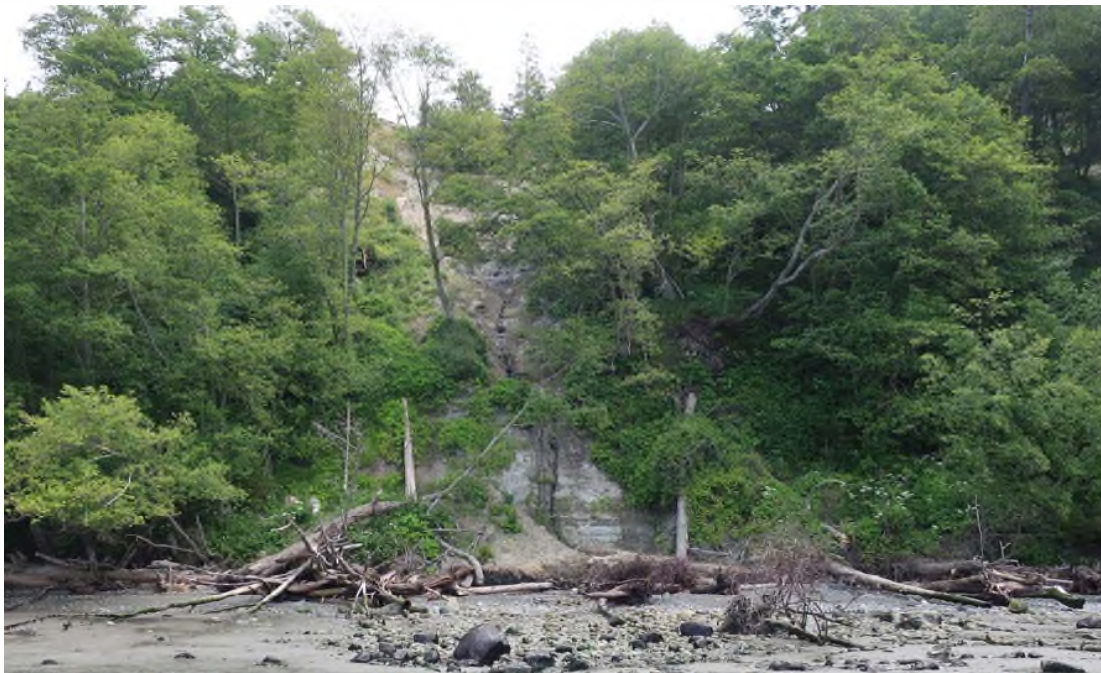
Another site where the sand unit collapse and flowed down over the hard silt/clay to the beach area below.
